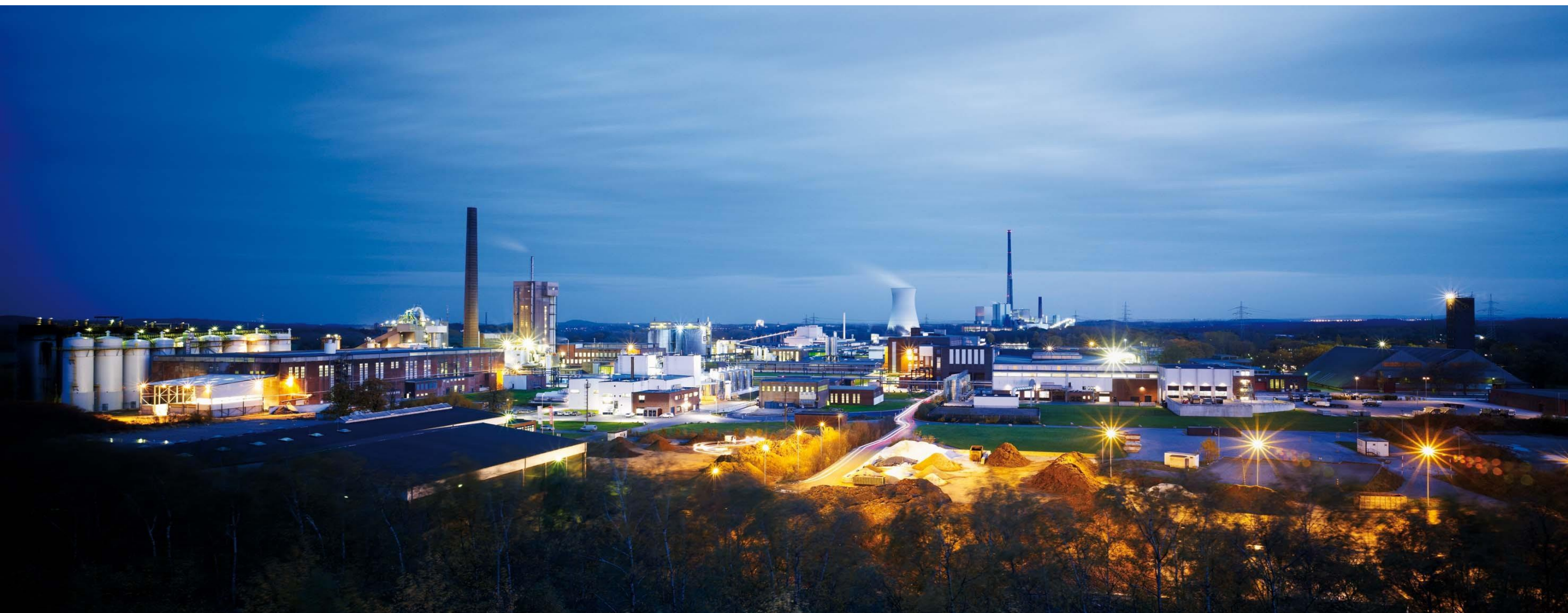
REMONDIS Headquarter – Lippewerk – Gemany
